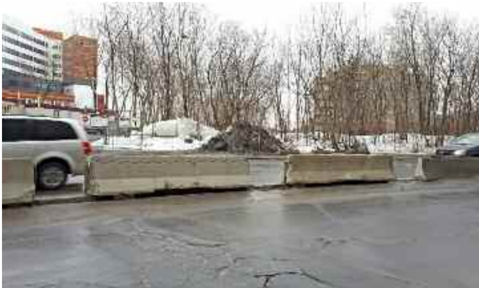
On February 16, the work seemed complete and the concrete barriers seemed loose from each other and the road surface.
