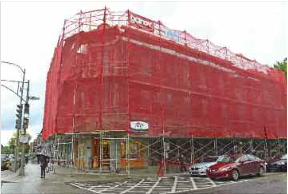
Scaffolding lined with red protective netting rises on the south side of Sherbrooke St. at Claremont Ave., where repairs to the brick façade of a building was taking place on September 7.
