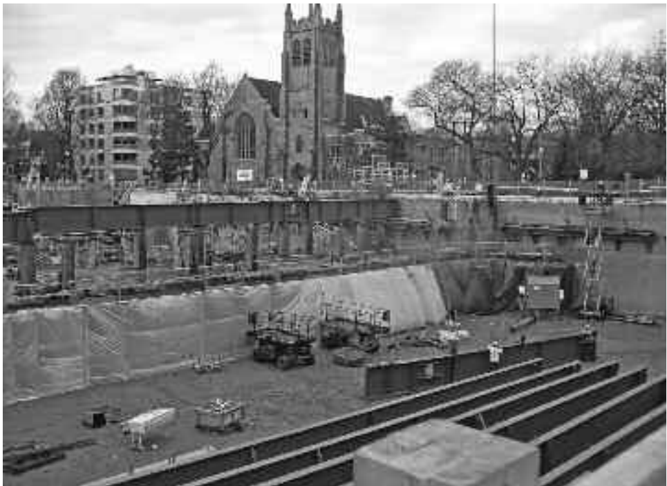
This is what the east rink looked like December 4, 2012, just before the steel beams (foreground) were lifted into place to support the green roof – published in the Independent December 11, 2012.
