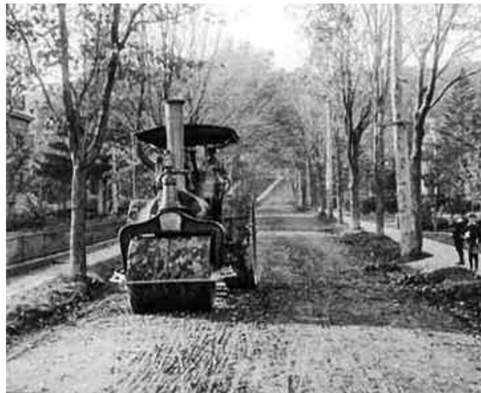
Rosemount being "macadamized" (paved), date unknown; 18 Rosemount is on far left. The source of the photo is the Westmount Historical Association archives, as published in The Westmount Historian , September 2009.
