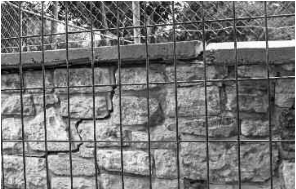
A closer look at the Belmont Cresc. wall, August 16, and a large crack that had formed.
