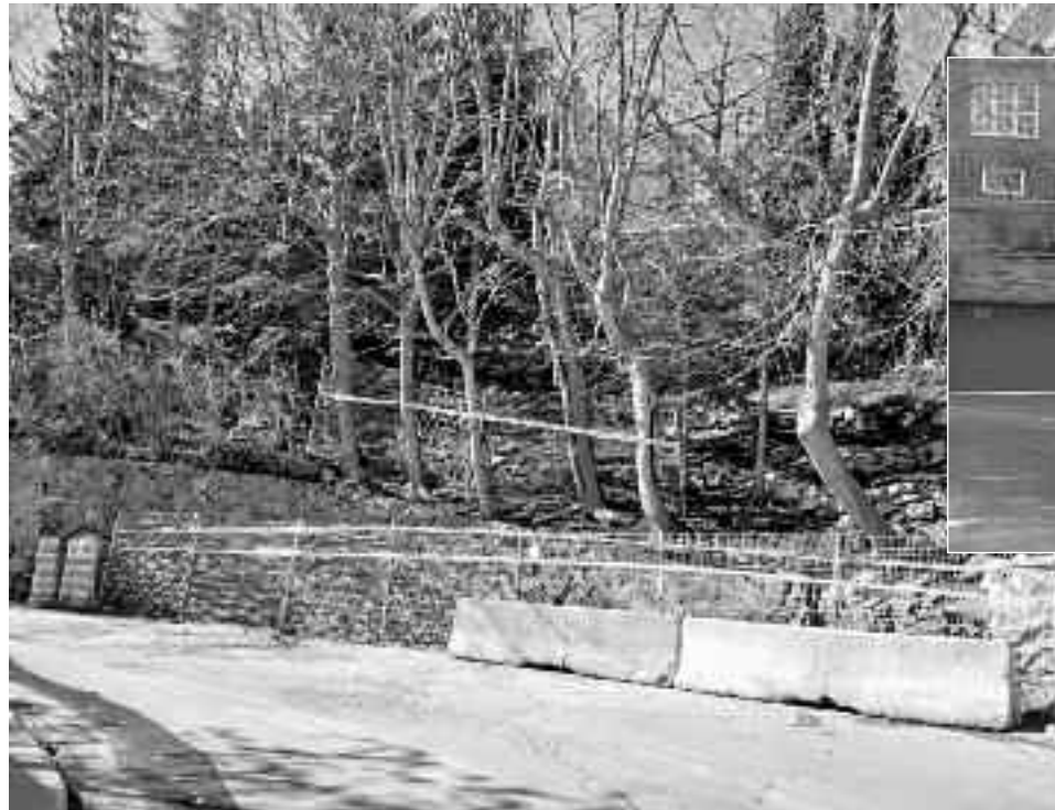
Jersey barriers and netting were installed on Belvedere March 29 to protect cars from rocks rolling downhill. Inset: Police cars block Belvedere Rd. at the Boulevard March 28.
