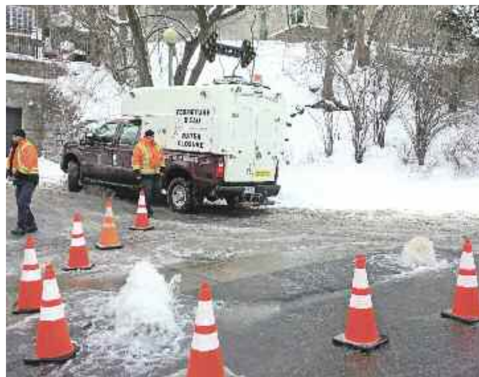
Crews repair a failed valve overnight January 18-19. Water is seen gushing out in two places on the Boulevard at Belvedere. Photo courtesy of Patrick Martin
