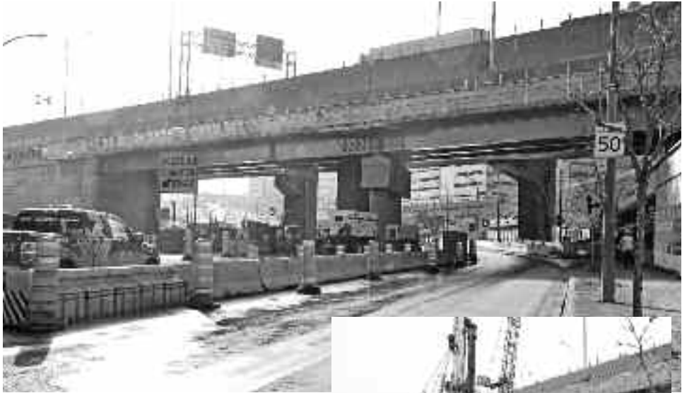
A glance at these two shots of St. Jacques St. just west of Glen Rd. (main photo was taken November 2, and inset April 6) reveals that, apart from the removal of heavy equipment, the eastbound elevated overpass (in the foreground), previously made of concrete, has been replaced with a framework of massive steel beams.
